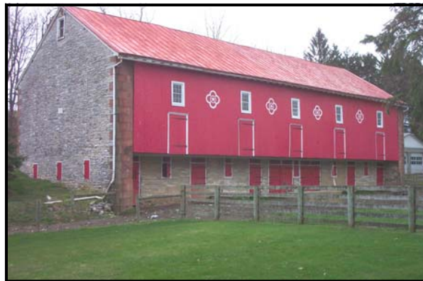
This barn was built in 1856 by Augustus and Matilda Leiss. It is located in the village of Host, Berks County.
